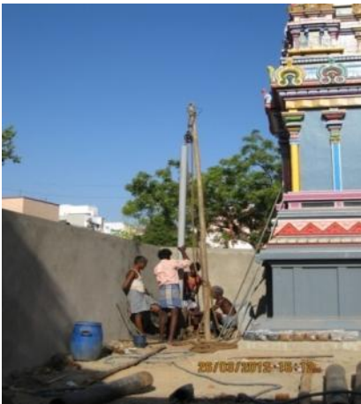
Restoration of temple tanks
