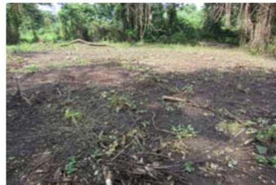
View (III) of allotted site after cleaning
